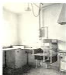
Built-in sinks in the kitchen
