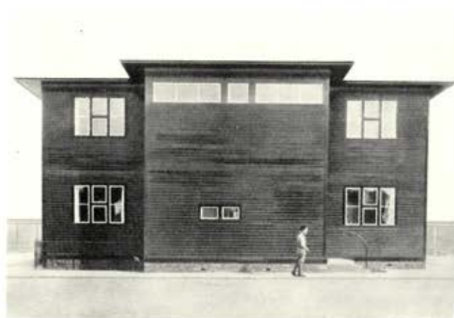
Rear view showing the staircase which is provided with external illumination.
